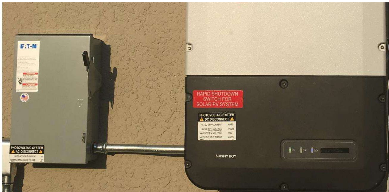
Figure 2: An example of the Sunny Boy US-41 inverter’s built-in DC disconnect switch labeled as the Rapid Shutdown Switch per NEC Article 690.56(C).
