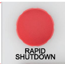
Figure 5.14 Inverter rapid shutdown and EPO initiation switch
