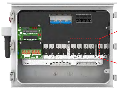
Figure 5.21 Battery cable connection
